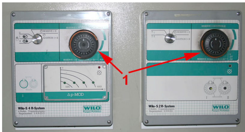
Figure 58: Controlling recirculation pumps using a time switch (1)
