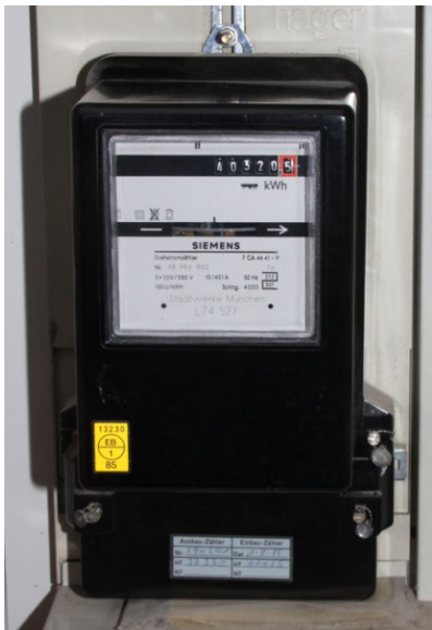
Analogue electricity meter with rotating disc (Ferraris)
