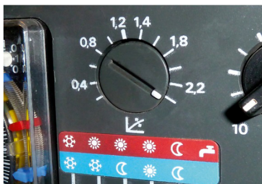
Figure 52: Setting the gradient of the heating curve on the heating controller. The setting for moving the curve in parallel is on the right.
