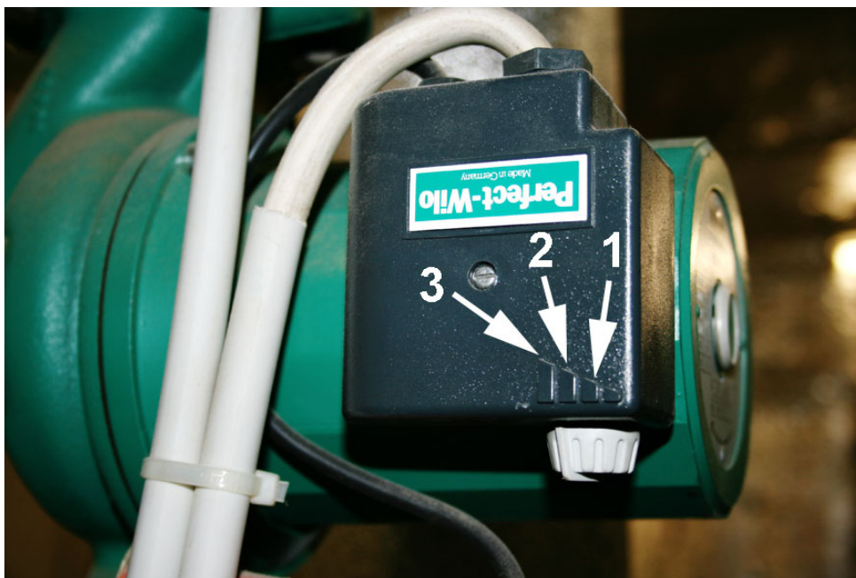
Figure 44: Recirculation pump with adjustable pump output
